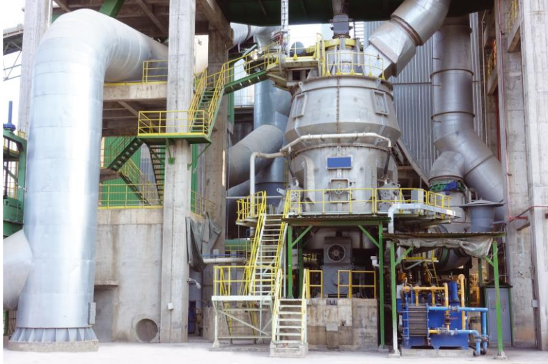
Figure 1. Vertical Cement Mill
